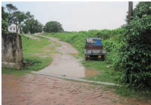
Broken compound wall of the ITI, Indranagar (Boys). Parking of private vehicle within the ITI campus area.
