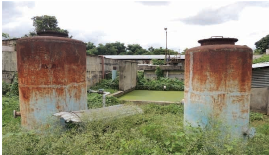
Non-functional liquid waste treatment plant at AGMC & GBP Hospital
