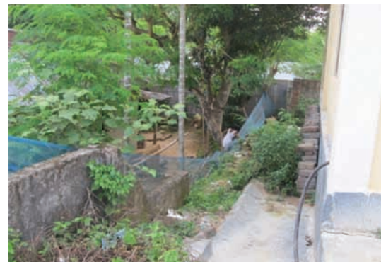
Broken compound wall of the ITI, Jatanbari in close proximity to a private household needed immediate reconstruction.
